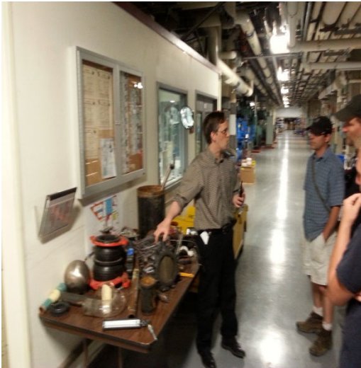
Seth the Facility Engineer explaining types of problems water can cause to the system ,constant monitoring and Maintenance are critical.
