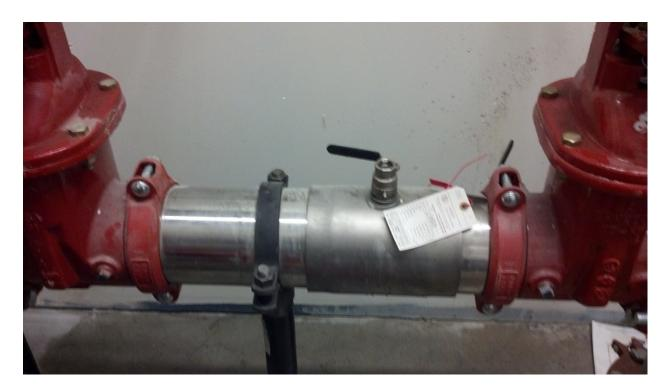
This is a 6" Ames/Colt 200 DCVA on a fire system. To access the internal checks, the outer sleeve is loosened and actually slides left. The bracing is mounted in concrete on the floor and even if the top of the bracket is removed, it is still not possible for this sliding action due to the bottom of the brace. The Watts 957 RP is designed the same way, and I suppose others. Needless to say, the placement of pipe supports are very important when these types of assemblies are installed.
