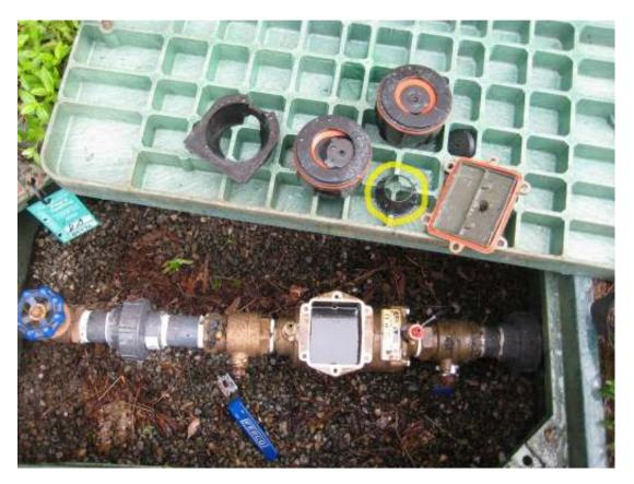
Attached is a photo of a 1.5" Febco 850 at the Costco #001 on 4<sup>th</sup> Ave. Both checks went right to 0 while testing.
